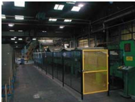
Blanket Press 2 Fence with interlocked gates
