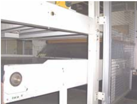
Rotary Shear 2, Conveyor diverting reject board to cage (different angle)
