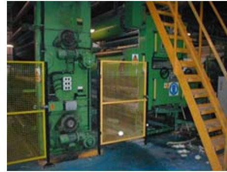
Double Backer Glue Unit 2 Interlocked Gates
