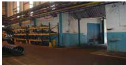
Risk Assessment Area
